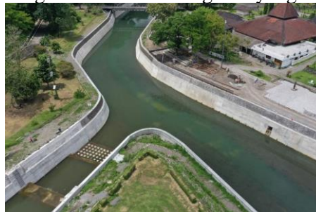
Gambar 1. Ground sill Sumber: Opak, 2022
